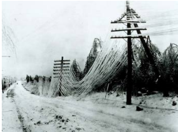
Figure 3: Due to added weight frozen cables are dragged much lower
